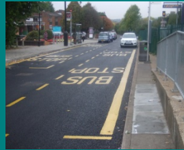
Castle Bar Park Station (Ealing) Implemented: Feb 2010 (£146k)
