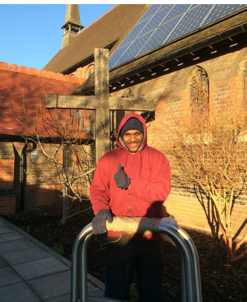
Cycle stand installation at St George's Church, Southall
