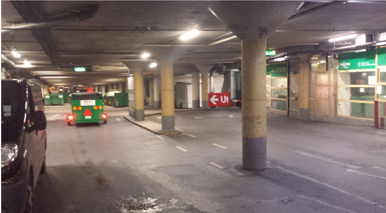
Old Town consolidation centre, Stockholm
